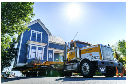
Built Environment Relocated Homes
